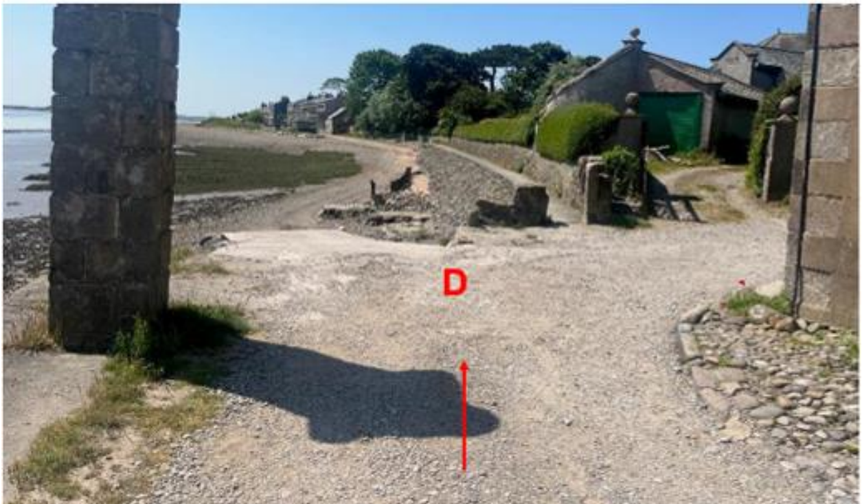
'Gate Pier' at point D:
